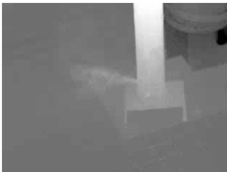
Leaks can pop up in unexpected locations, such as in this pipe support.
