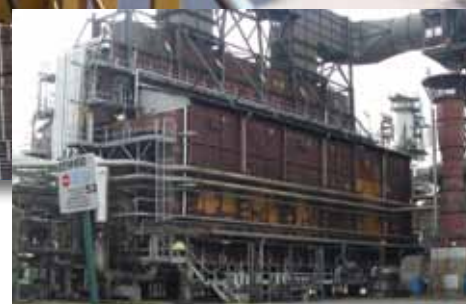
Petroval inspected this crude distillation unit furnace.
