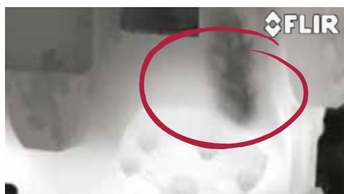
Captured gas leak.
