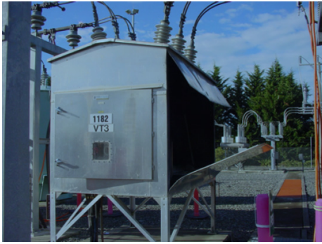
Circuit Breaker with Panels Blown Off
