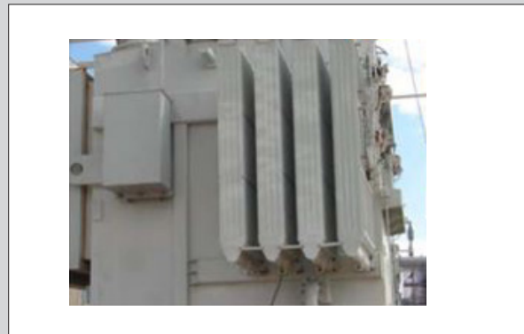
Closed Radiator Flapper Valve
